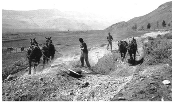
Photo: B.C. Archives Construction of an irrigation system at Walhachin for orchards, 1910.
