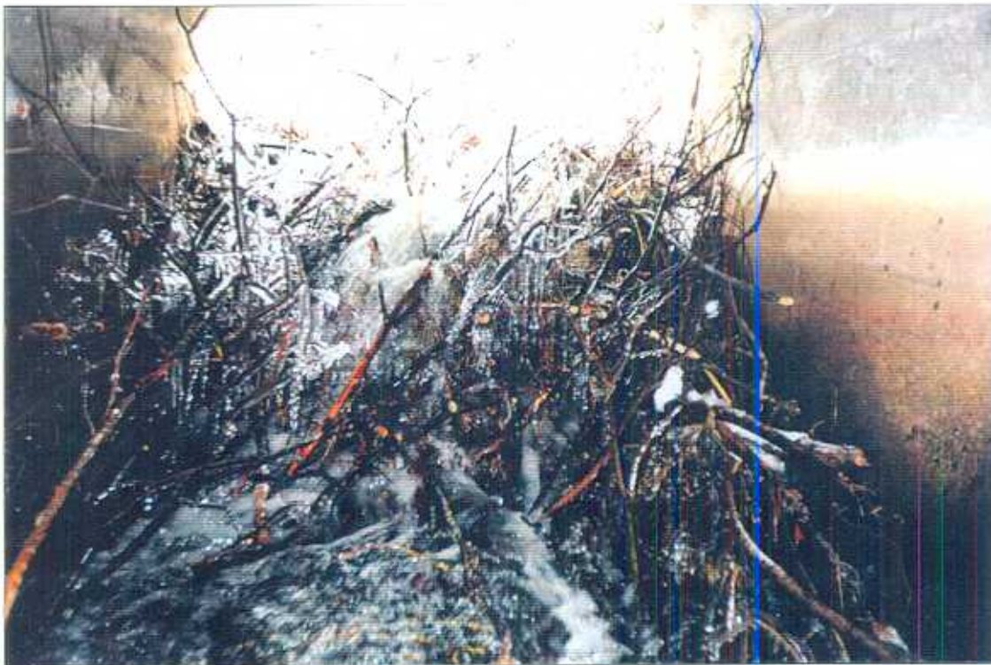
Photo 8. Beaver dam partially blocking the upstream end of the culvert, upstream view from within the culvert. Stream Name: Hydraulic Creek Site #: 18 Reach #: 4 GPS Coordinates: 49°47'75N 119°12'04W Code: Fb•D•N•2
