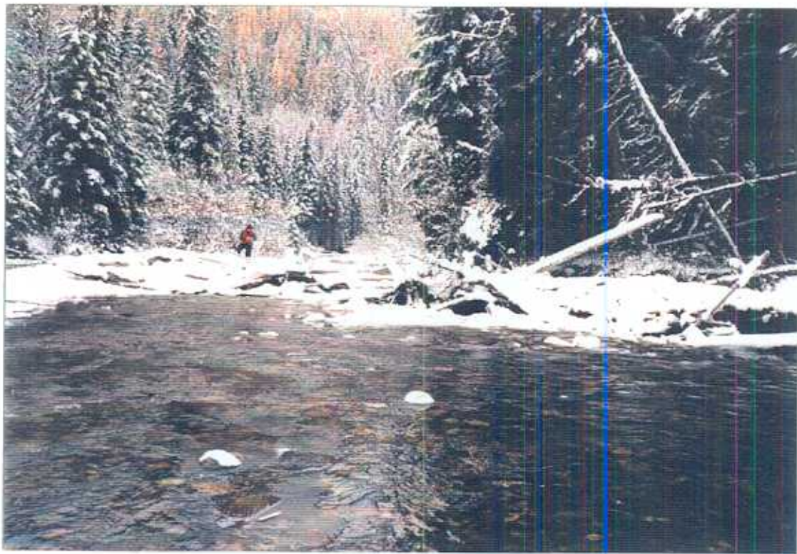
Photo 16. Debris jam blocking a side channel u/s from weir structures, downstream view. Stream Name: Mission Creek Site #: 43 Reach #: 7 GPS Coordinates: 49°52'22N 119°05'64W Code: Fb•D•N/F•1
