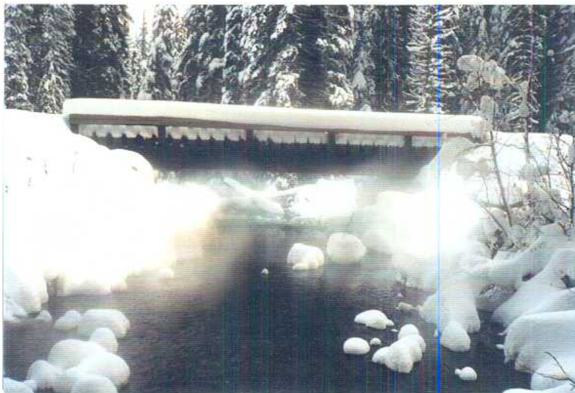
Photo 5. Bridge crossing with sufficient vertical & horizontal clearance, downstream view. Stream Name: Belgo Creek Site #: 20 Reach #: 3 GPS Coordinates: 49°??'??N 119°04'36W Code: Q-C-F-3
