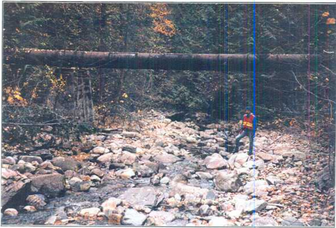
Photo 3. Non-functional water pipe crossing over the channel, downstream view. Stream Name: Klo Creek Site #: 4 Reach #: 2 GPS Coordinates: 49°49'56N 119°21'95W Code: N/A
